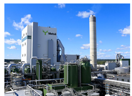
New Äänekoski Plant commissioned in 2017
