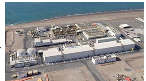
Seawater Desalination Plant
