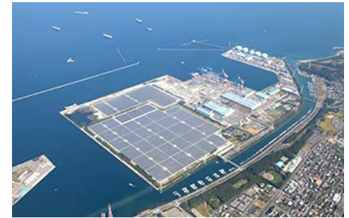
Oita-Hiyoshibaru Solar Power Plant
