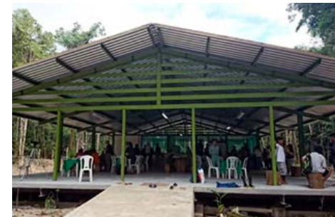
Completed Field Station
