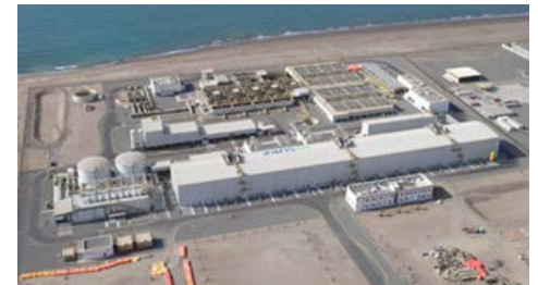
Seawater Desalination Plant
