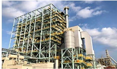
Ichihara Biomass Power Plant
