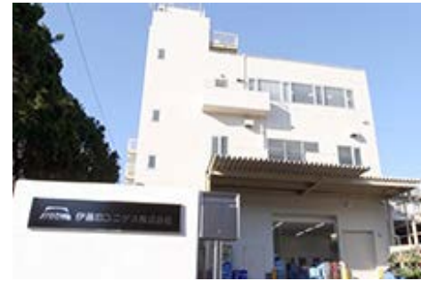
New offices of ITOCHU Uneedus Co., Ltd. (Tsuzuki Ward, Yokohama)
