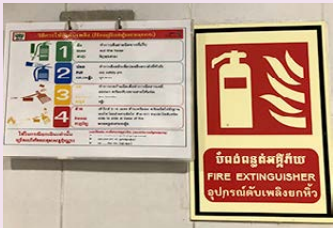
All Signs in Cambodian on Fire Prevention Facilities
