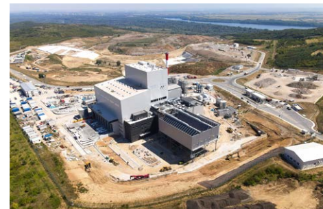
Serbia/Belgrade Waste Management Public-Private Partnership project (under construction with Interim Service)
