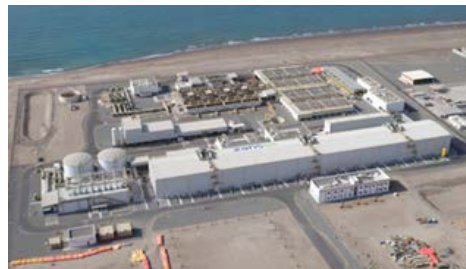
Seawater Desalination Plant
