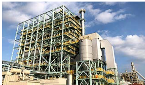
Ichihara Biomass Power Plant
