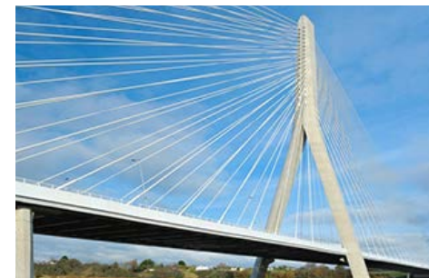
Structure Made with Blast Furnace Slag
