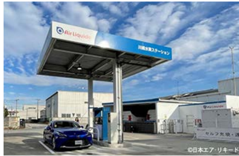
Hydrogen Station (Kawasaki Hydrogen Station of Air Liquide Japan G.K.)
