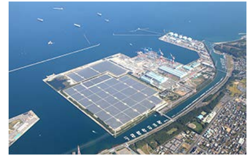
Oita-Hiyoshibaru Solar Power Plant
