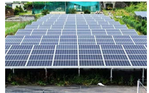
Clean Energy Connect Off-site Distributed Power Supply
