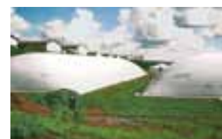
Image of the finished hog farm methane project
