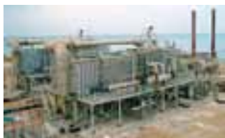
Desalination facilities under construction (Saudi Arabia)
