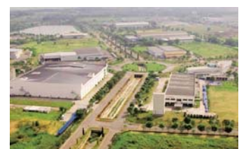
Karawang Industrial Park
