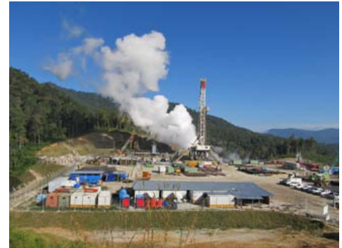
Drilling site of geothermal well
