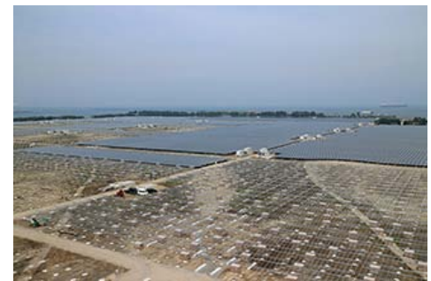
Steady progress of construction at the Oita Large-Scale Solar power plant
