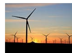
Shepherds Flat wind power plant
