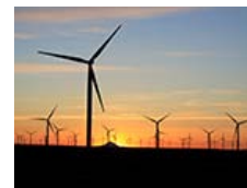
Shepherds Flat wind power plant
