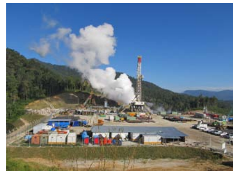
Drilling site of geothermal well
