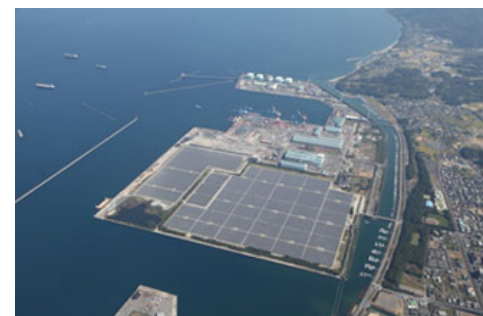
Panoramic view of the Oita Hiyoshibaru Mega-Solar Power Plant
