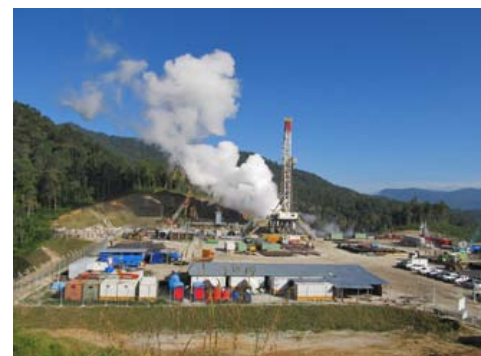
Drilling site of geothermal well
