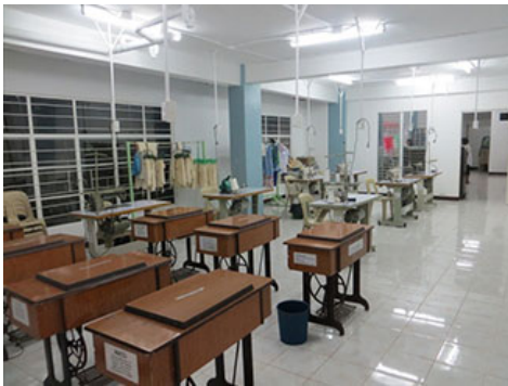
The renovated basement room of sewing machines
