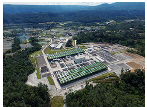
The first unit of the Sarulla Geothermal IPP Project
