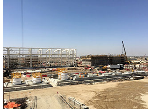
Seawater desalination plant (under construction)
