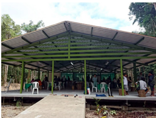
The completed Field Station
