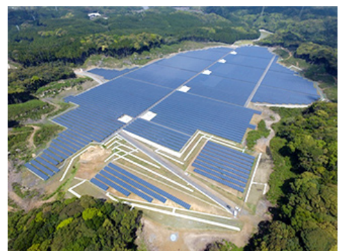
the Saga-Ouchi Solar Power Plant
