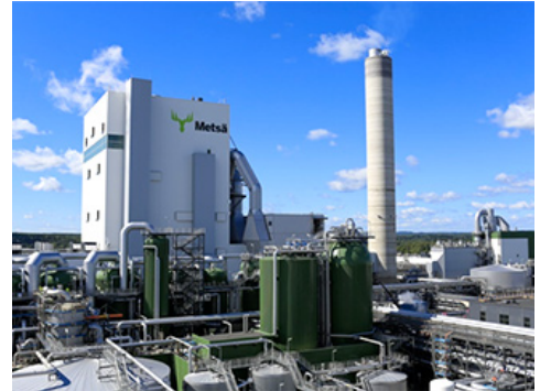
Äänekoski Mill, a new mill that began operating in 2017
