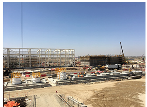
Seawater desalination plant (under construction)
