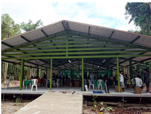
The completed Field Station
