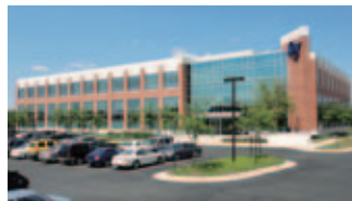
Headquarters of U.S. N.E.W. Customer Services, Inc.
