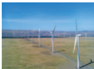
Shepherds Flat power plant
