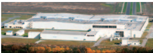
Exterior view of YOKOHAMA R.P.Z. factory
