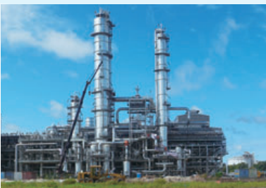
Brunei methanol production project
