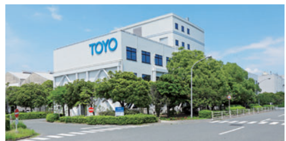
Toyo Advanced Technologies' headquarters
