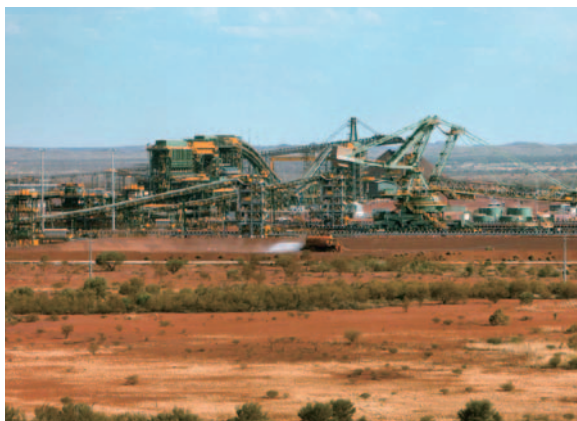
Ore processing facilities at the Jimblebar Iron Ore Mine (photo provided by BHP Billiton)
