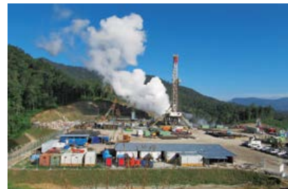
Project construction site
