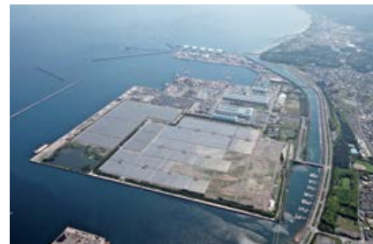
Oita Hiyoshibaru Mega-Solar Power Plant
