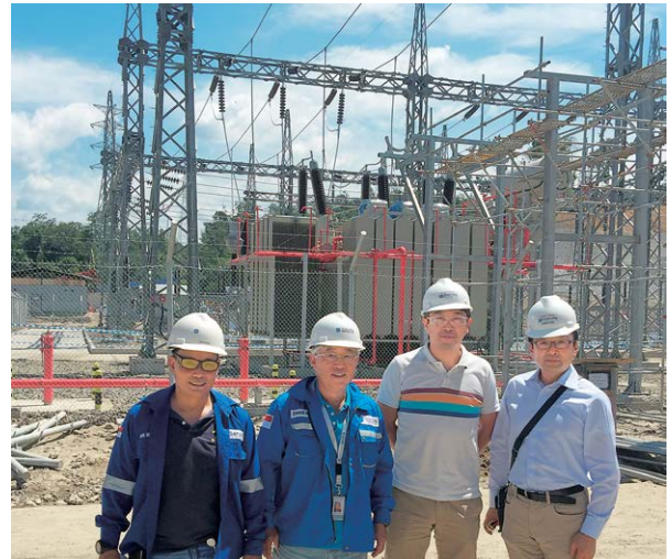
Visiting employees posted to work on the construction site of one of the world's largest geothermal power plants, in Sumatra, Indonesia
