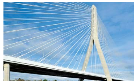
Structure employing blast furnace slag
