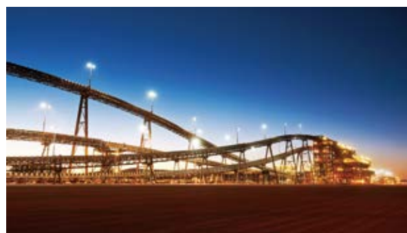
WAIO's Ore Processing Plant (Photo courtesy of BHP)
