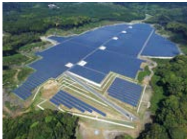
Saga-Ouchi Solar Power Station, Japan
