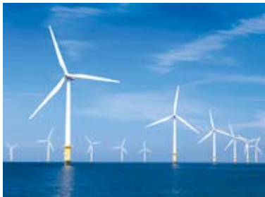
Butendiek Offshore Wind Power Plant, Germany
