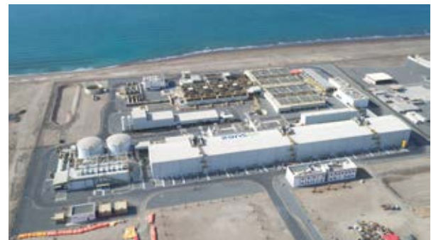
Barka Seawater Desalination Plant in Oman
