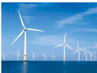
Butendiek Offshore Wind Power Plant, Germany
