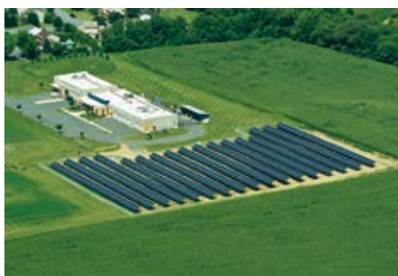
Nazareth Solar Power Facility in Pennsylvania, USA
