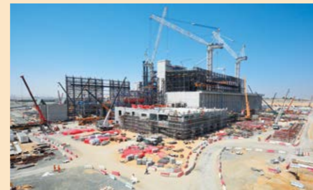
Progress of the construction of an energy-from-waste plant in Dubai
