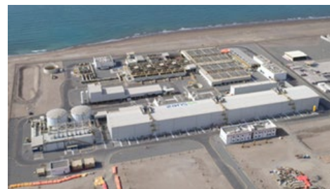
Seawater Desalination Plant
