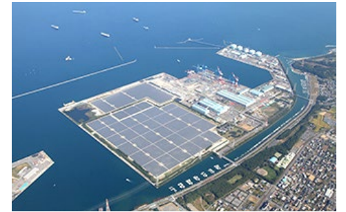
Oita-Hiyoshibaru Solar Power Plant
