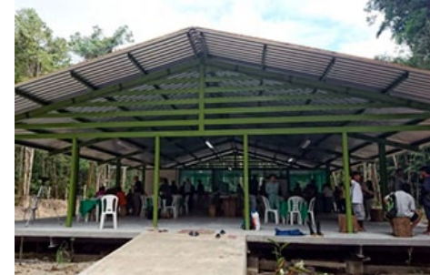
Completed Field Station
