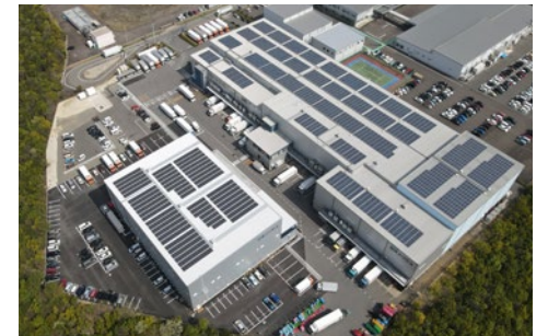
i GRID SOLUTIONS On-site Distributed Power Supply
