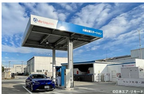
Hydrogen Station (Kawasaki Hydrogen Station of Air Liquide Japan G.K.)
