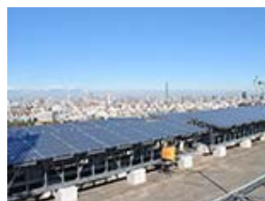
The solar panel installed on the roof of ITOCHU Corporation's Tokyo Head Office building
