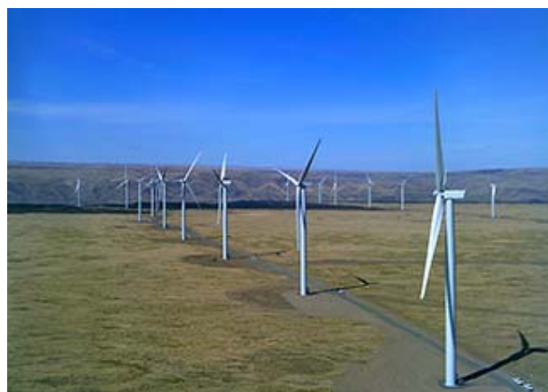
Shepherds Flat power plant
