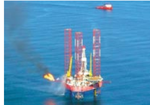
Oil field development platform in Sakhalin
