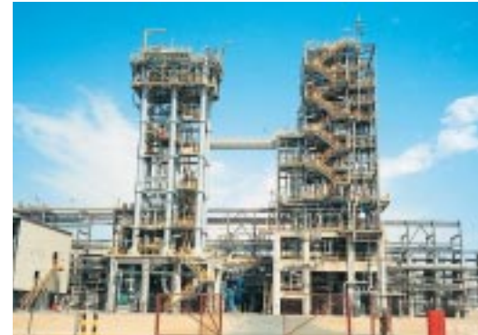
Polypropylene plant in Turkmenistan
