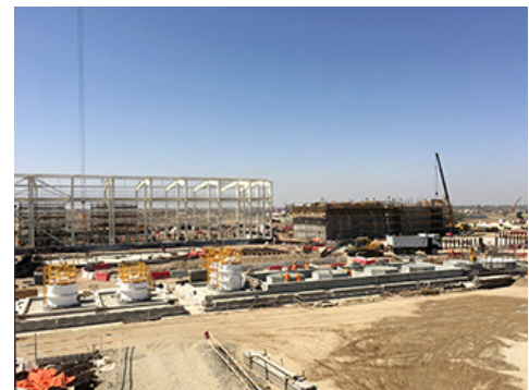
Seawater Desalination Plant (During Construction)
