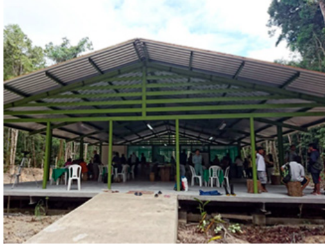
Completed Field Station
