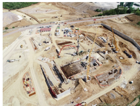
Construction site for energy-from-waste facility, Belgrade, Republic of Serbia.
