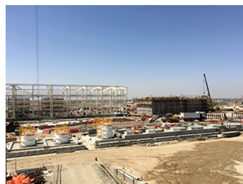
Seawater Desalination Plant (During Construction)
