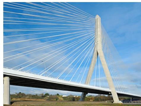
Structure Made with Blast Furnace Slag
