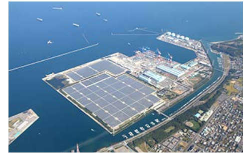
Oita-Hiyoshibaru Solar Power Plant
