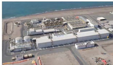
Seawater Desalination Plant
