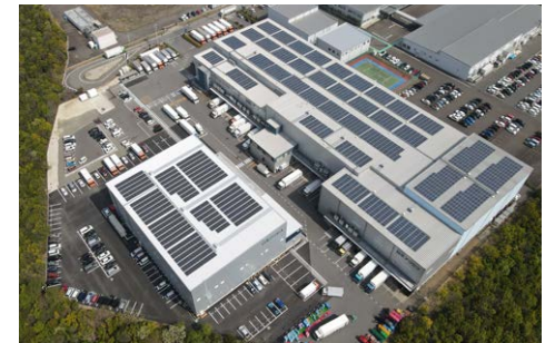
i GRID SOLUTIONS On-site Distributed Power Supply
