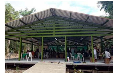
Completed Field Station
