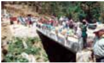
A small bridge connecting Guatemala's communities
