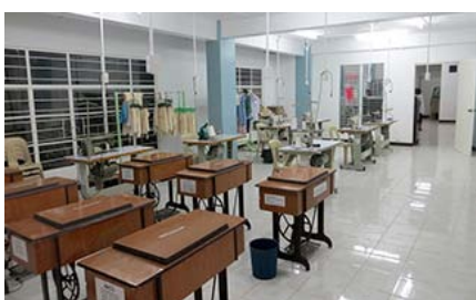
The renovated basement room of sewing machines
