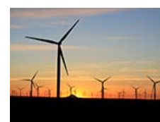
Shepherds Flat wind power plant
