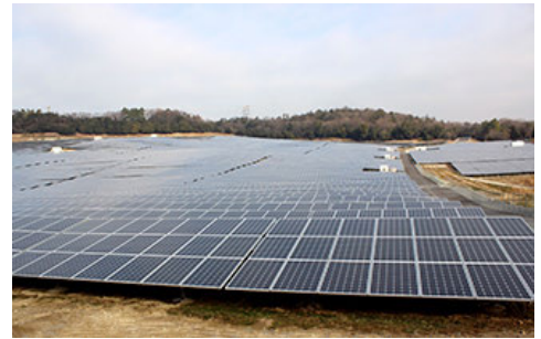
Shin-Okayama Mega-Solar Power Plant
