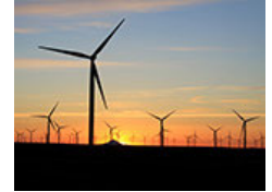
Shepherds Flat wind power plant
