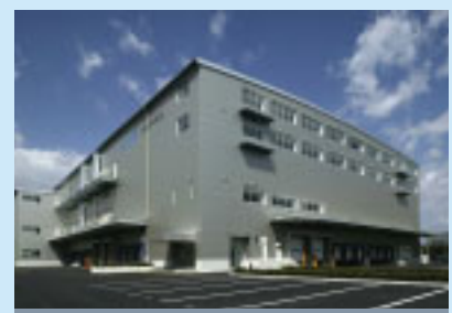
A distribution center of NIPPON ACCESS INC.
