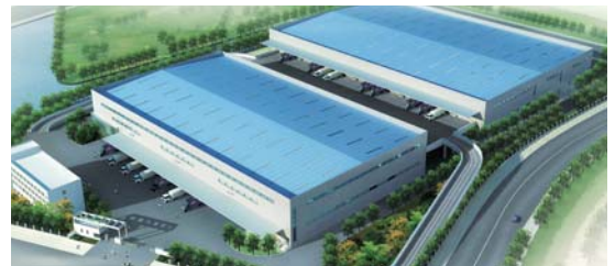
Shanghai Anting logistics center of ITOCHU LOGISTICS (CHINA) CO., LTD.
