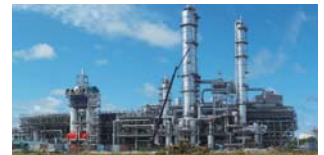
Methanol Plant in Brunei (Manufacture of methanol)
