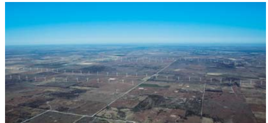
Keenan II power plant
