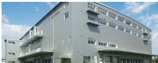
NIPPON ACCESS chilled distribution center
