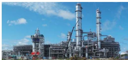
Exterior view of plant
