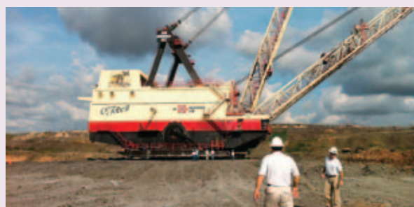
Dragline operation for overburden removal
