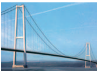
Image of İzmit Bay Bridge
