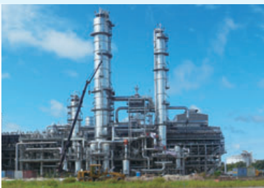
Brunei methanol production project
