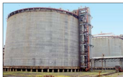
LPG storage facilities in Mumbai (photo courtesy of Aegis)
