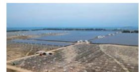
Site of the future Oita mega-solar facility
