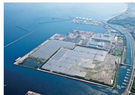
Oita Hiyoshibaru Mega-Solar Power Plant (commenced commercial operation in March 2016)
