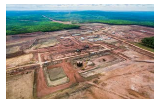
Construction site of a crude oil processing facility
