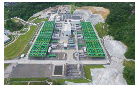
The first unit of the Sarulla Geothermal IPP Project
