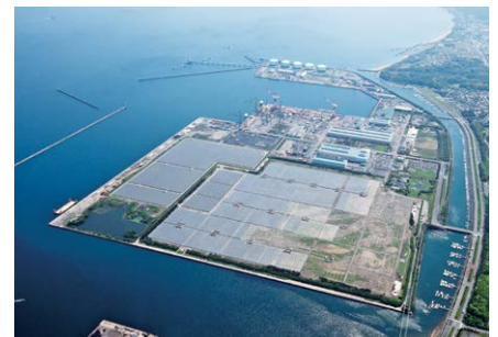
Oita Hiyoshibaru Mega-Solar Power Plant (commenced commercial operation in March 2016)
