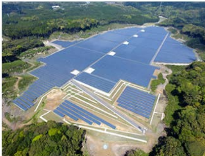
Saga-Ouchi Solar Power Plant
