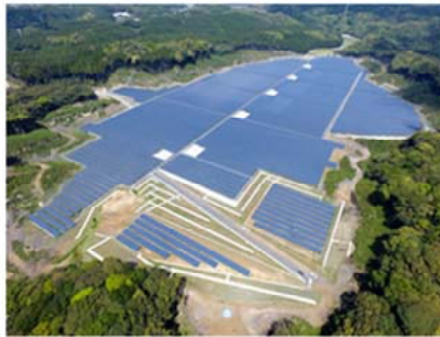
Saga-Ouchi Solar Power Plant
