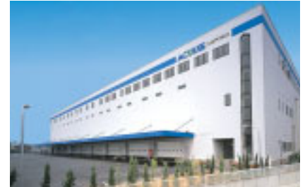
YUKIJIRUSHI ACCESS' multi-temperature distribution center
