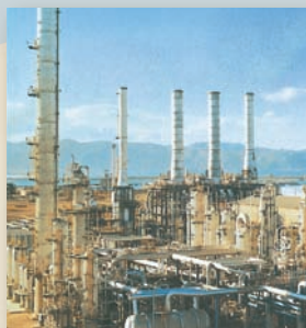
Petrochemical complex constructed in Algeria
