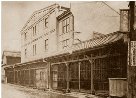
Japan's first reinforced concrete warehouse, built by Chubei Itoh II
