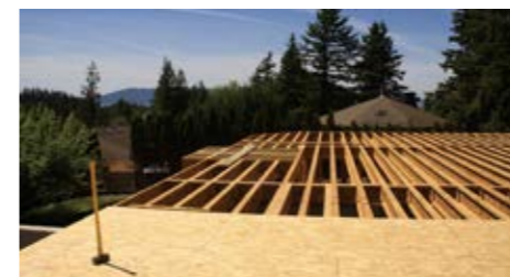
Engineered wood products made of laminated veneer lumber manufactured by Pacific Woodtech Corporation
