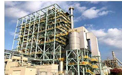
Exterior of Ichihara Biomass Power Plant
