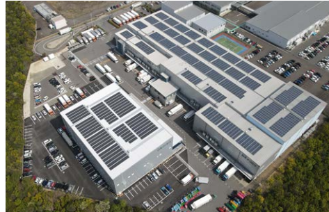
On-site Distributed Power Supply Operated by i GRID SOLUTIONS
