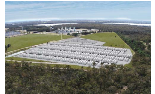
An Image of Akaysha’s Project under Development in Australia.
