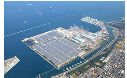
Oita-Hiyoshibaru Solar Power Plant
