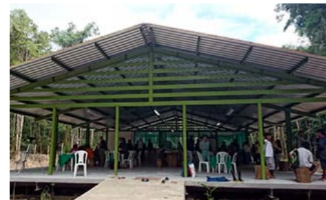
Completed Field Station
