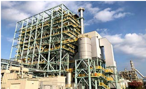
Exterior of Ichihara Biomass Power Plant
