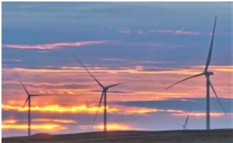
Bowman Wind Power Plant in North Dakota
