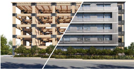
ITOCHU women's dormitory built with timber construction
