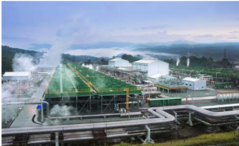
Sarulla Geothermal Power Plant (2nd/3rd Unit)
