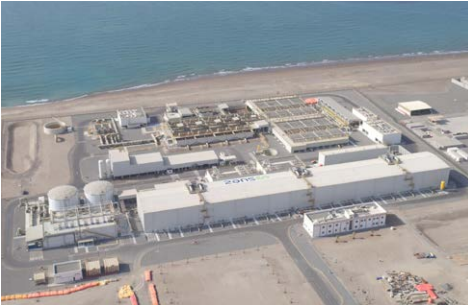
Aerial view of Oman seawater desalination plant
