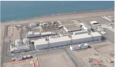
Aerial view of Oman seawater desalination plant
