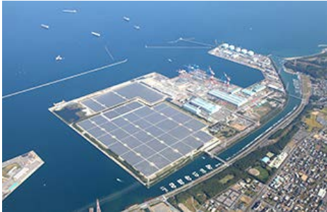
Oita-Hiyoshibaru solar power plant
