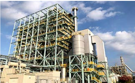
Exterior of Ichihara Biomass Power Plant
