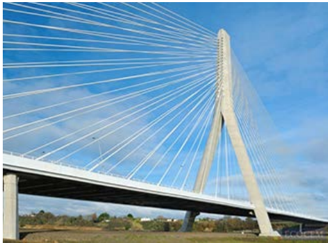
Structure made with blast furnace slag
